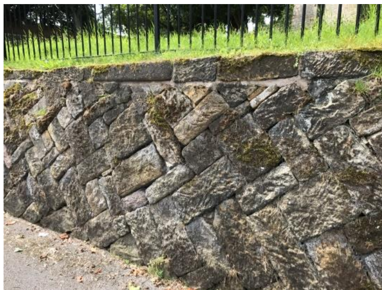
Figure 16 Local sandstone walling with courses of blocks laid in herringbone fashion (© Steve Austin)
